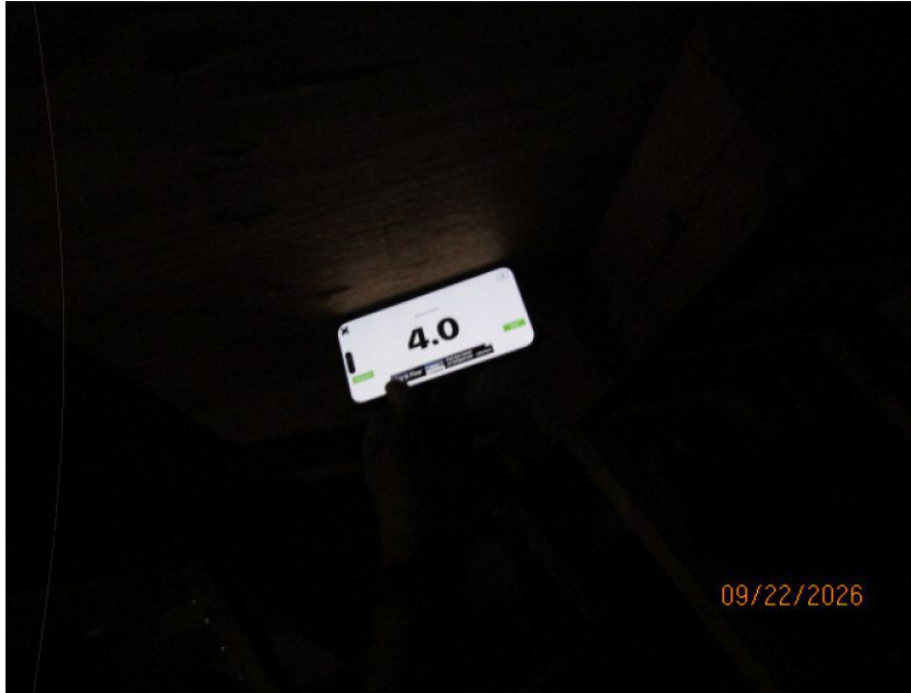
Primary Slope Measurement, Covering 100% of Main Roof
