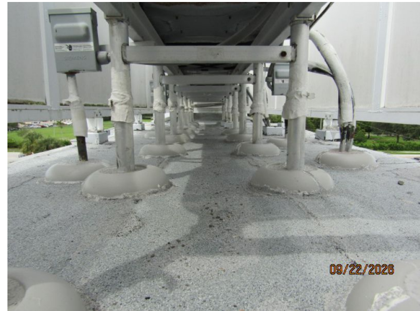
Built Up/Rolled Asphalt (Flat) Roof Covering
