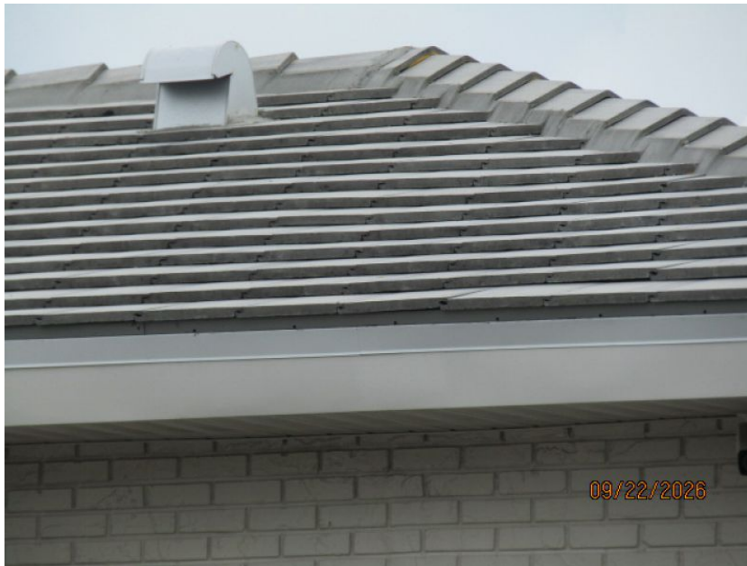
Concrete/Clay Tile Roof Covering
