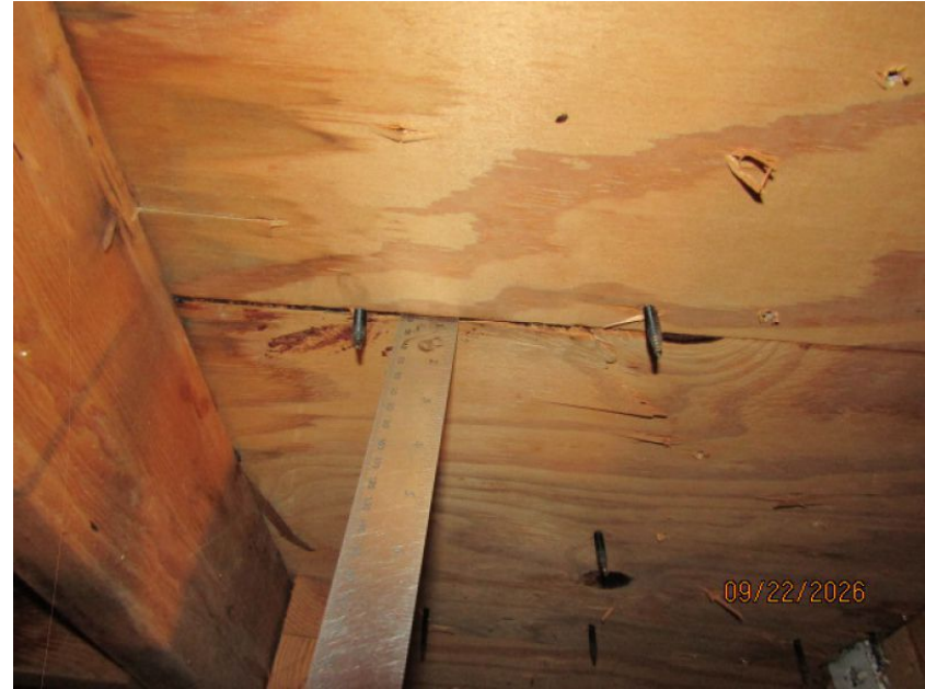
5/8" Deck Thickness Confirmed
