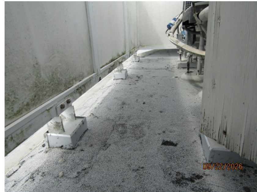
Built Up/Rolled Asphalt (Flat) Roof Covering
