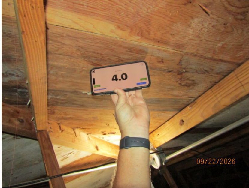
Primary Slope Measurement, Covering 100% of Main Roof
