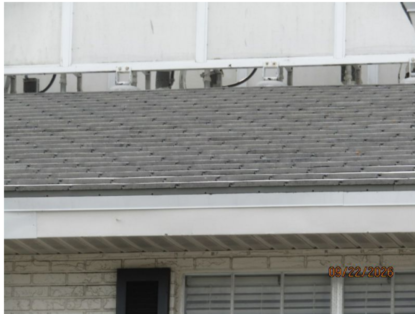
Concrete/Clay Tile Roof Covering
