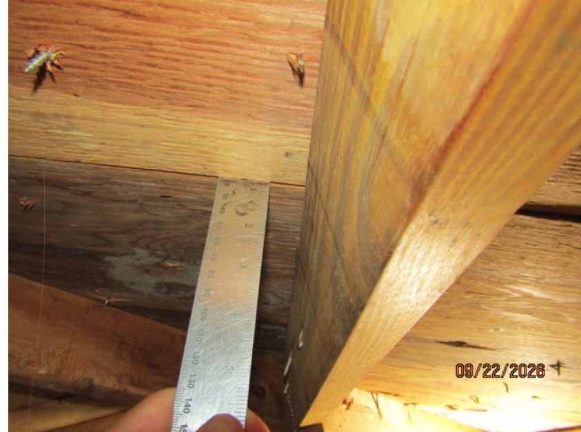
5/8" Deck Thickness Confirmed
